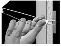
Snap straps at wall by pushing side to side, snapping of straps level with flange of cap.
