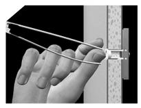
Snap straps at wall by pushing side to side, snapping of straps level with flange of cap.
