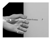
A Drill 1/2" diameter hole. Hold metal channel flat alongside plastic straps and slide channel through hole.
